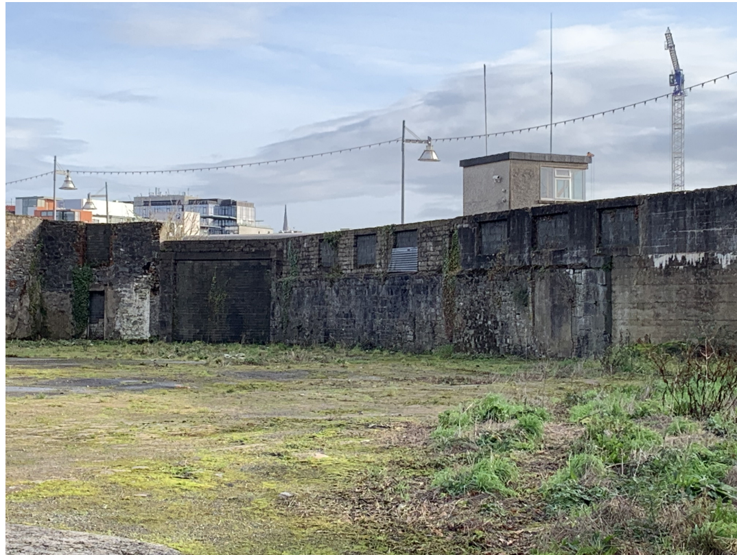
03- Image of existing Shipyard site
