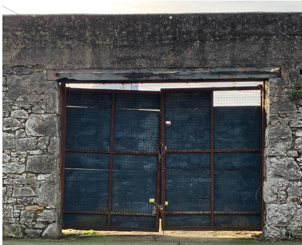
01- Image of existing gate to Shipyard site
