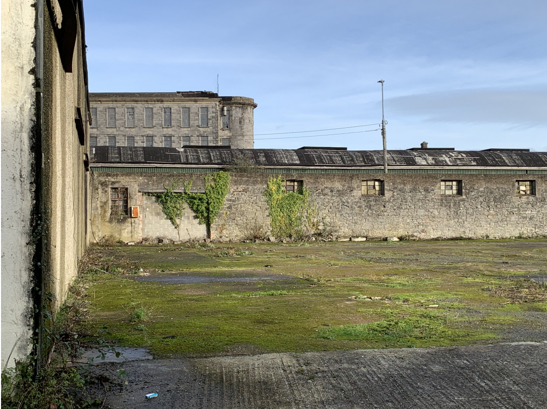
02- Image of existing Shipyard site
